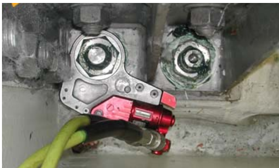
XLCT-2 with SW 65 in tight struts
