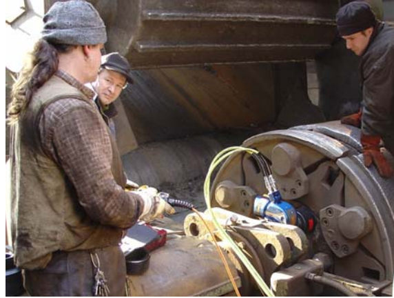
MXT-10 being used on a scrap press
